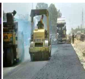
A road under construction
